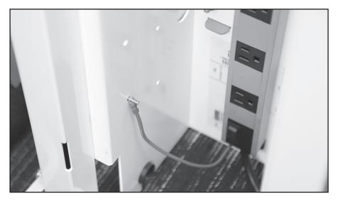
1. Place small screw into bottom hole on side of spine and slide on ground wire.
