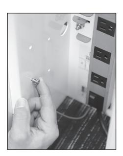
2. Place nut on screw and tighten the ground wire onto the side of the spine.
